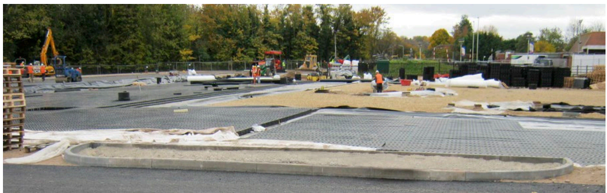
Attenuation/Retention, 4-8 modules in height = 20-40 cm
